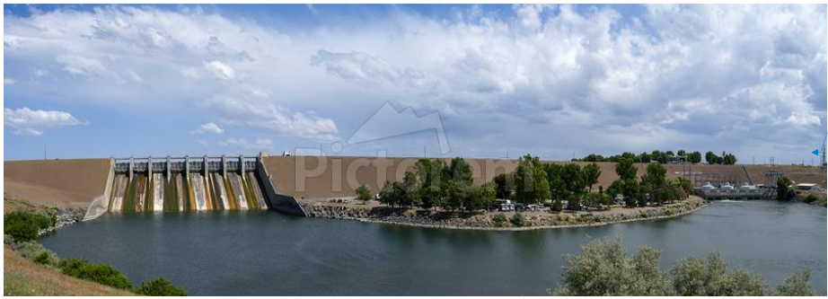
CJ Strike Dam and Spillway
