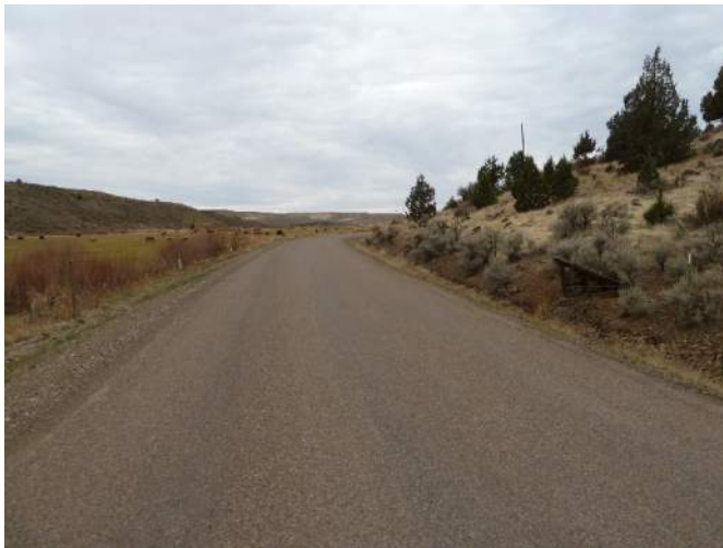
FIGURE 1 – TYPICAL COLD MIX ASPHALT ROAD (PLEASANT VALLEY RD)
