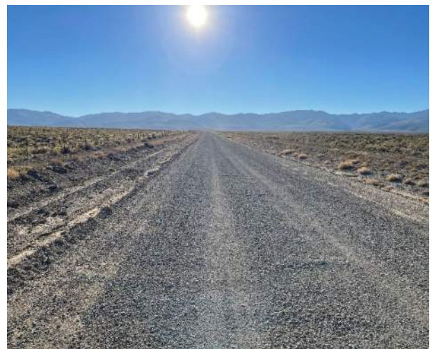
FIGURE 2 – TYPICAL GRAVEL ROAD (BACHMAN GRADE RD)
